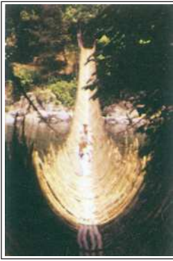
Figure 6.7: Rope Bridge (Arunachal Pradesh)
