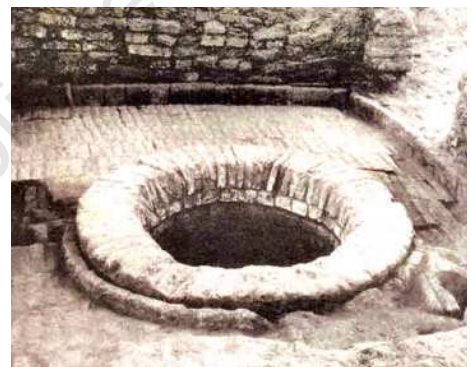
Top: A street in Mohenjo-daro with a drain. Above: A well.
