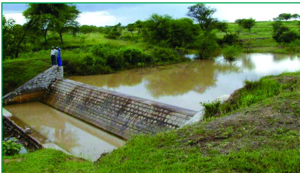
fig-1: Communitybased masonry dam
